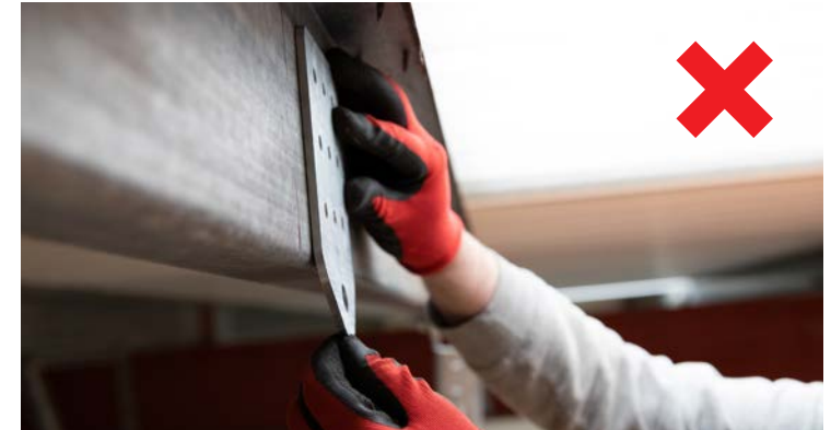
Fig. 1: Incorrect - bracket bends towards you
