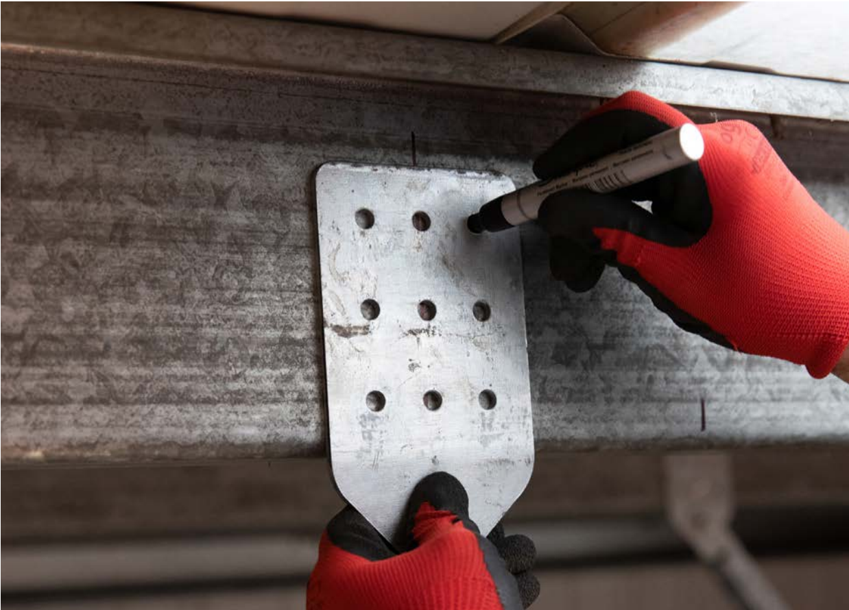
Fig. 1: Incorrect - bracket bends towards you
